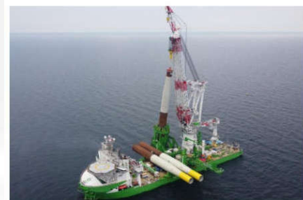
DEME "Orion" installing 360ft long piles weighing over 2,000T with its 5,000T crane and tailor-made motion compensated pile handling system
