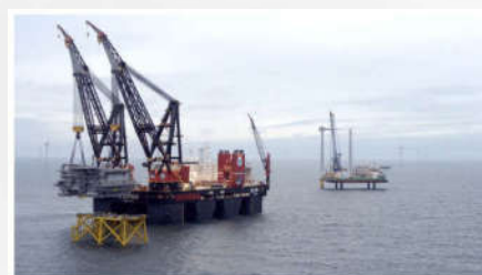
SMC "Sleipner" installing a substation using its twin 10,000T cranes in tandem
